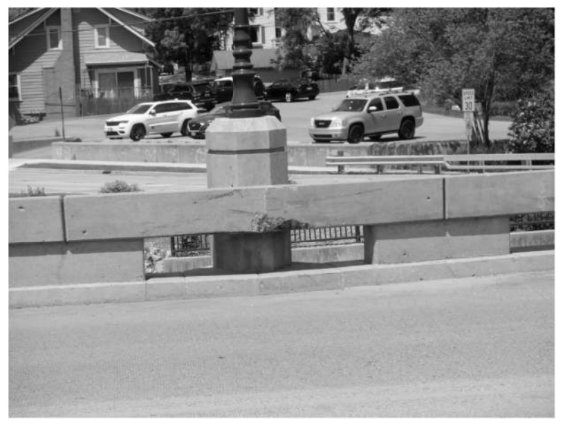
PHOTO 1 (North Parapet Elevation at Pier 7, Looking Northeast)
