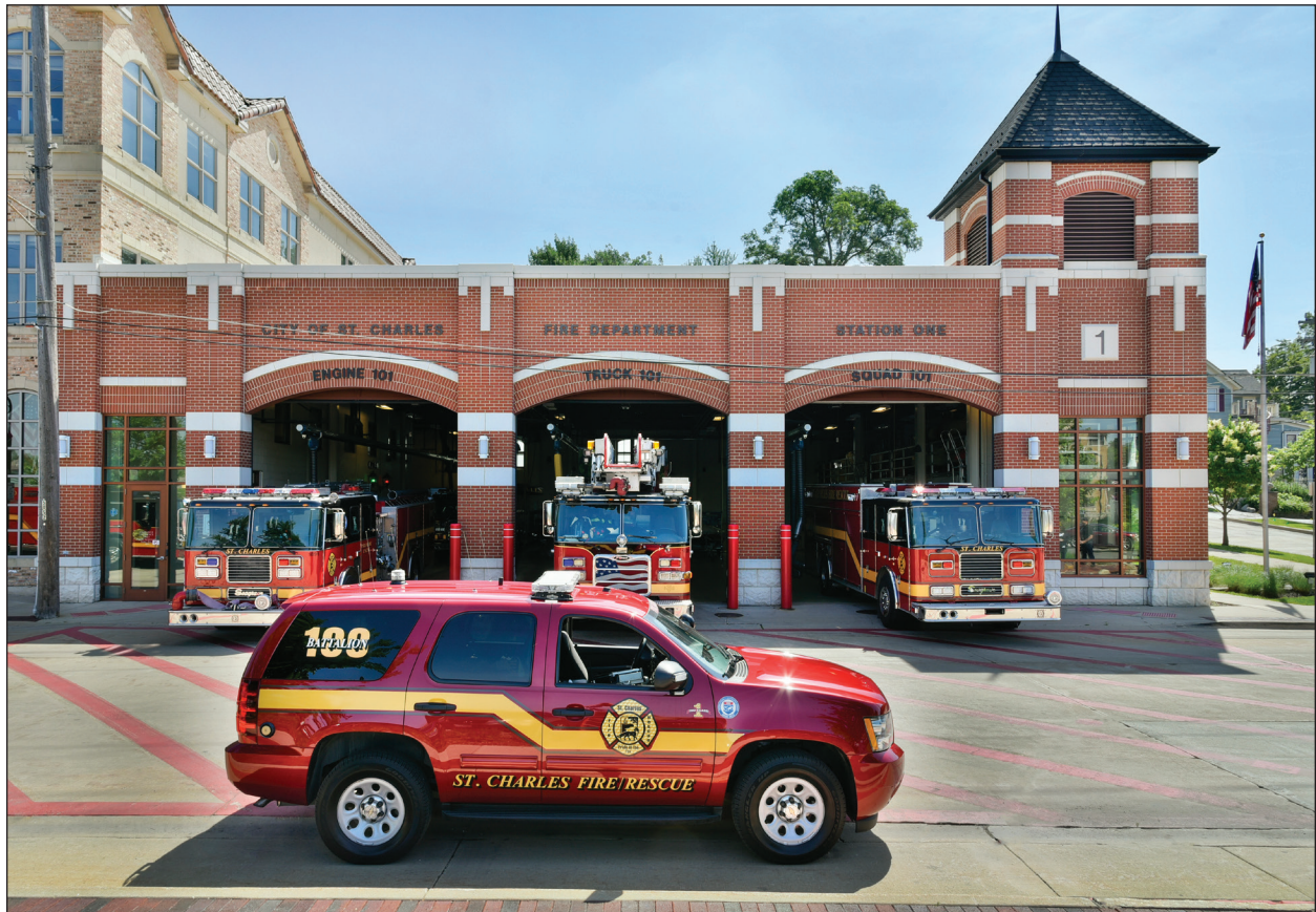
Fire Station #1 - 112 N. Riverside Ave. Central Station - Downtown Truck 101-Engine 101-Battalion 100
