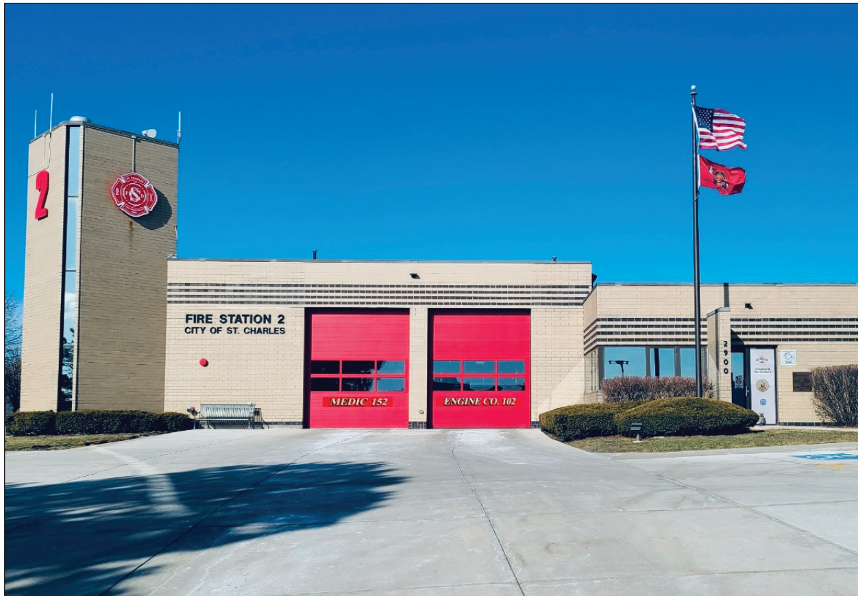
Fire Station #2 - 2900 Production Drive East Side
