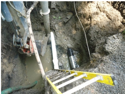
Figure 1 - Force Main Repair Clamp
